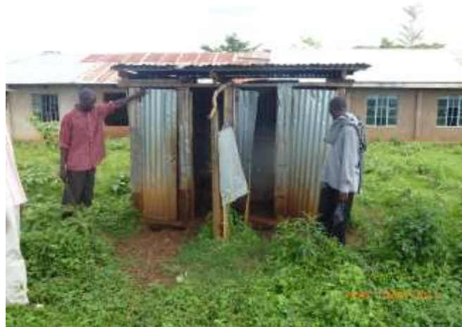
Existing Toilet block at Kubar Primary School
