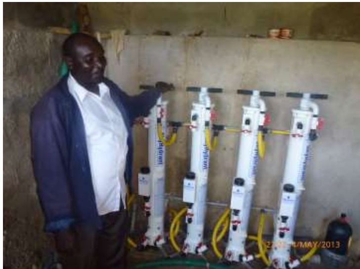
SkyHydrant Filters at Gona Dam, similar to those proposed for Manyasi Dam
