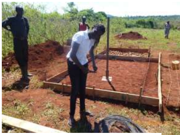
Wilfreda cutting tie wire for steel reinforcing within the concrete slabs
